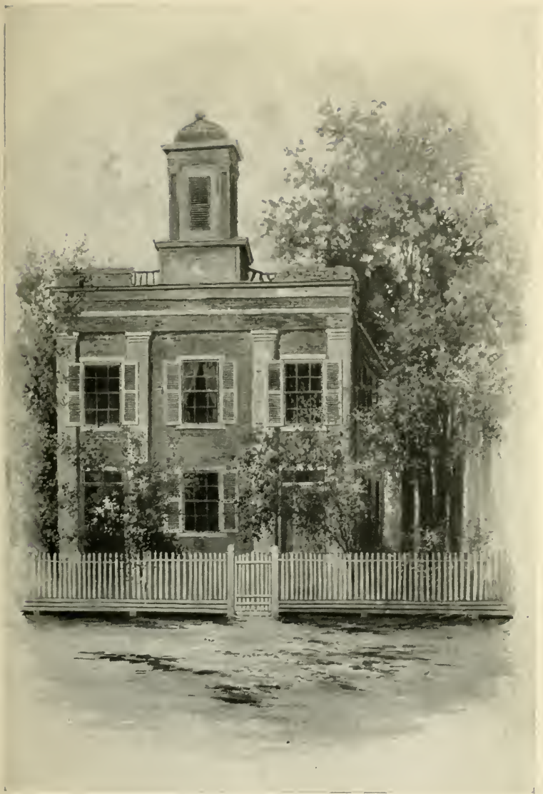
OLD SEMINARY HOMESTEAD, GREENFIELD—THE "CROW'S NEST." The center window on the second floor was where the Poet worked
